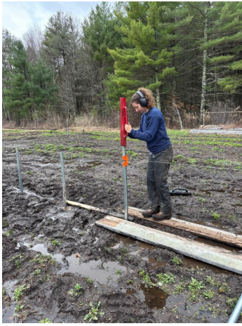
Determining location of posts
