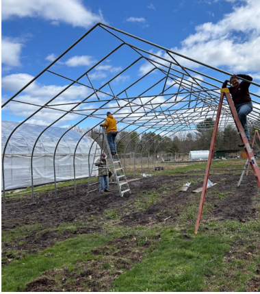
Getting the sides onto the new high tunnel!
