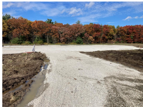
The bed area being filled and tamped with gravel, prior to bed construction
